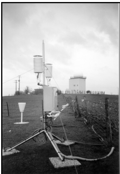
Photo 2 : Weather station and rain gauge installed 100 meters from the radar
